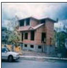
Figure 1: Typical two-story house in Canada (WHE Report 82)
