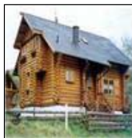
Figure 2: Typical log house in the Russian Federation (WHE Report 56)
