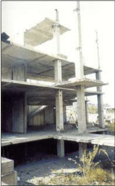
Figure 10: A lift-slab building of "Seria KUB" under construction (WHE Report 39, Kyrgyzstan)
