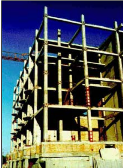
Figure 16: Seismic strengthening of precast columns with steel straps (WHE Report 66, Uzbekistan)
