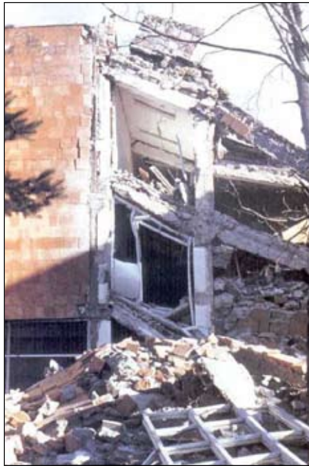
Figure 14: Building collapse in the 1988 Spitak (Armenia) earthquake (WHE Report 66, Uzbekistan)
