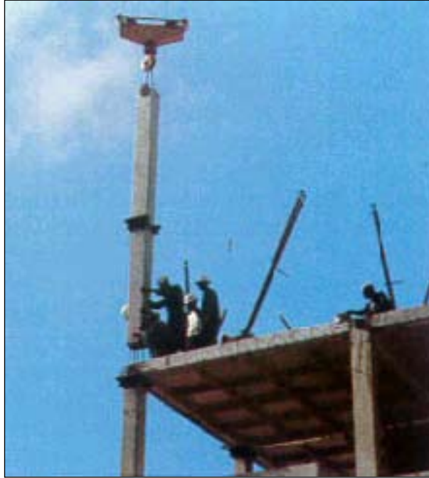
Figure 13: Assembly of precast columns in progress (WHE Report 68, Serbia and Montenegro)
