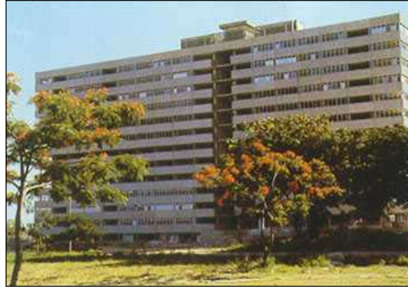
Figure 2: A typical precast slab-column building (WHE Report 68, Serbia and Montenegro)
