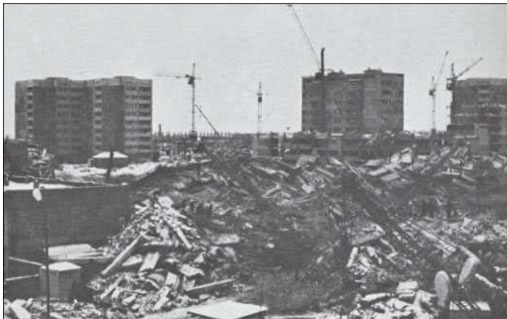
Figure 15: Large-panel concrete buildings remained undamaged in the 1988 Spitak (Armenia) earthquake (far back), whereas the precast frame buildings suffered extensive damage (foreground) 3 (WHE Report 32, Kazakhstan)
