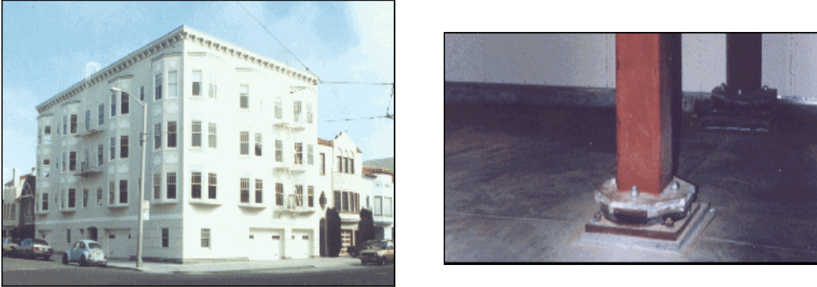
Figure 10: Marina apartment building (left); installation of FPS bearing at the column base (right)
