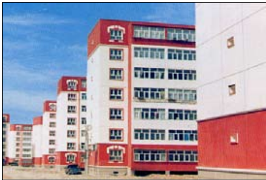
Figure 1: Base-isolated brick masonry building with RC concrete floors and roof in China (WHE Report 9)
