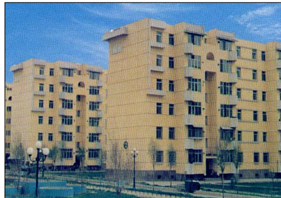
Figure 9: Base-isolated, brick masonry buildings remain undamaged in the 1996 Yunan earthquake (M 7.0) (WHE Report 9, China)
